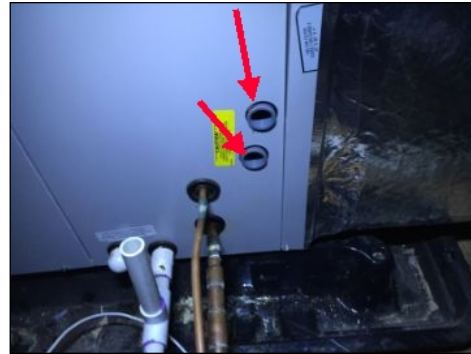
There are open ports drawing in air which should be plugged.
